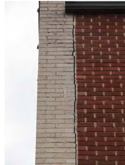
Open vertical seam between red and yellow brick
