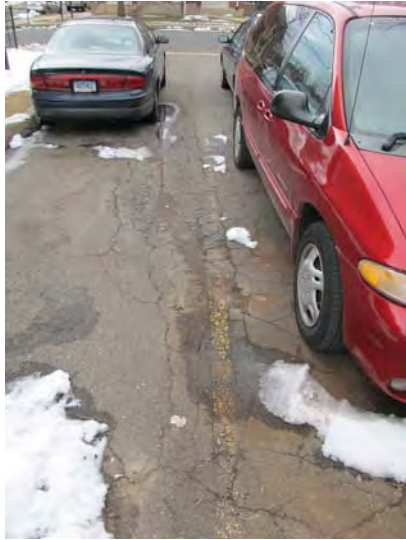
Asphalt paving at parking areas exhibits age-related cracks and deterioration
