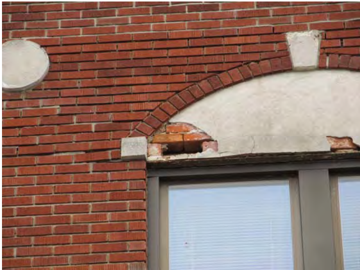
Area of brick and mortar loss at third floor level of Martin Street elevation
