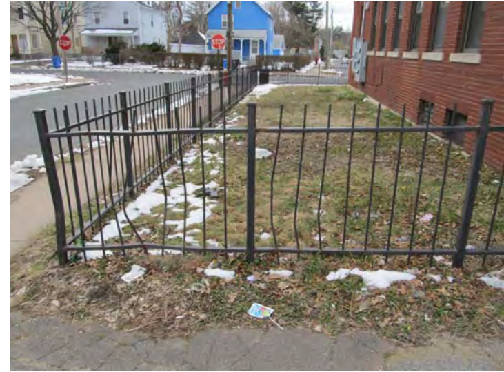
Wrought iron fencing along property lines at public streets is in need of minor repairs, surface prep, and painting
