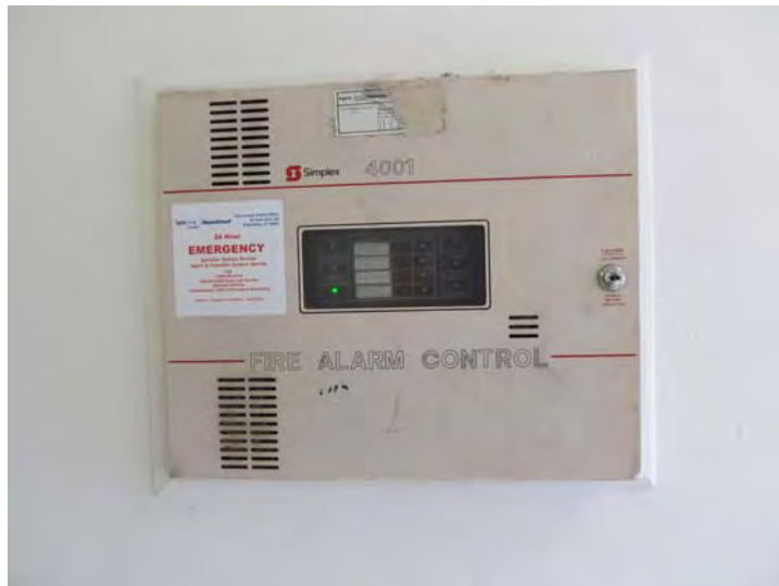
Original zone-type fire alarm control is serviceable but at or near the end of its expected useful service life
