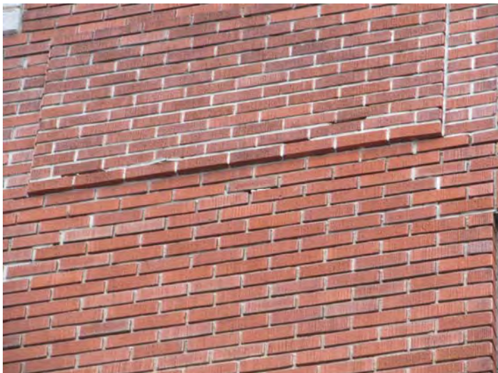
Select areas of mortar loss evident at various other locations around building
