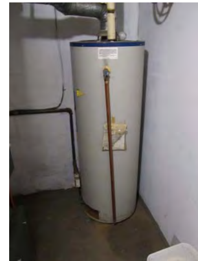
Domestic hot water tank for former laundry room – Laundry room not in place at present time and tank not being used
