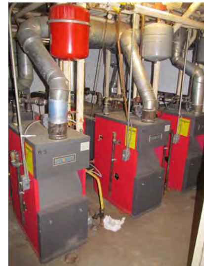
New combination boilers/domestic hot water generators were recently installed for all units in a basement-level mechanical room
